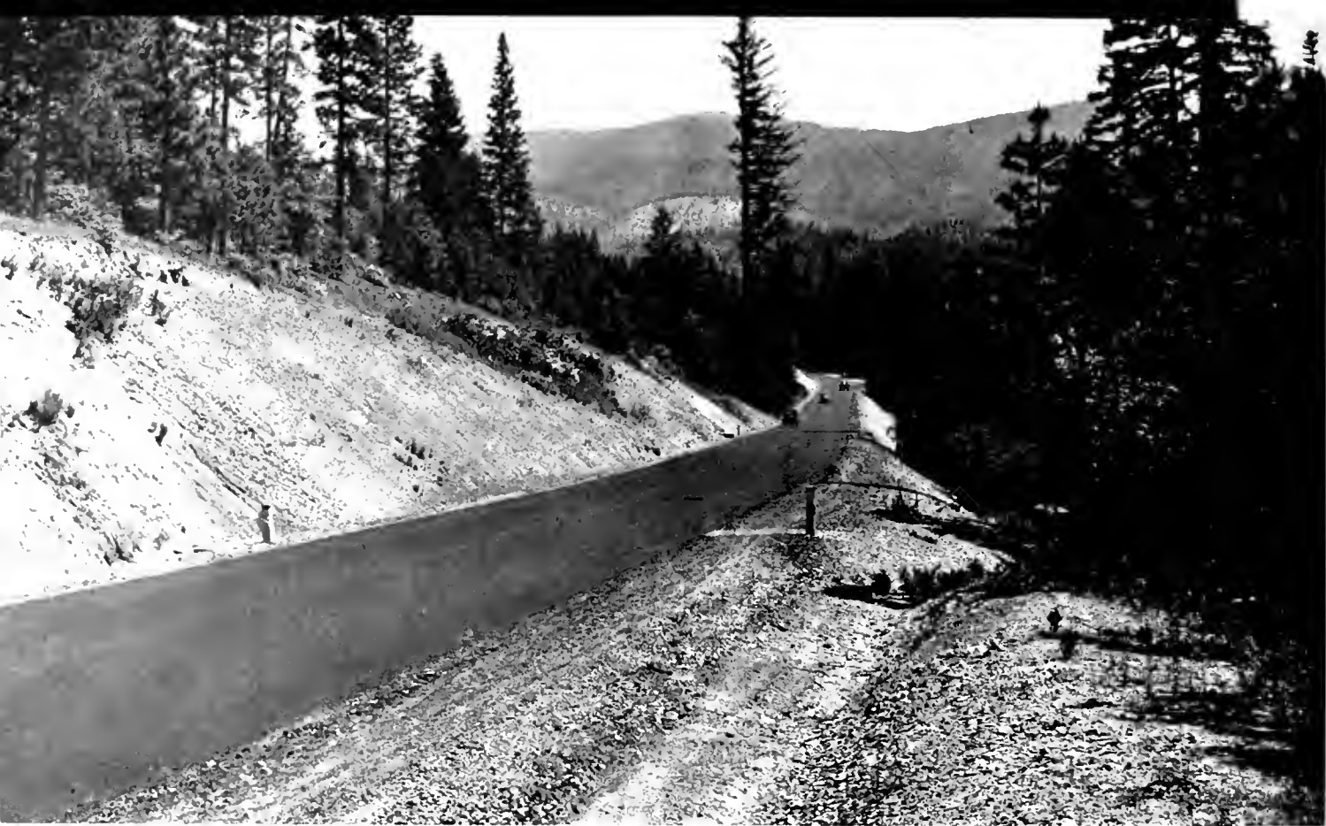
View of completed surface on the Feather River Highway in scenic region between Howells and Keddie
